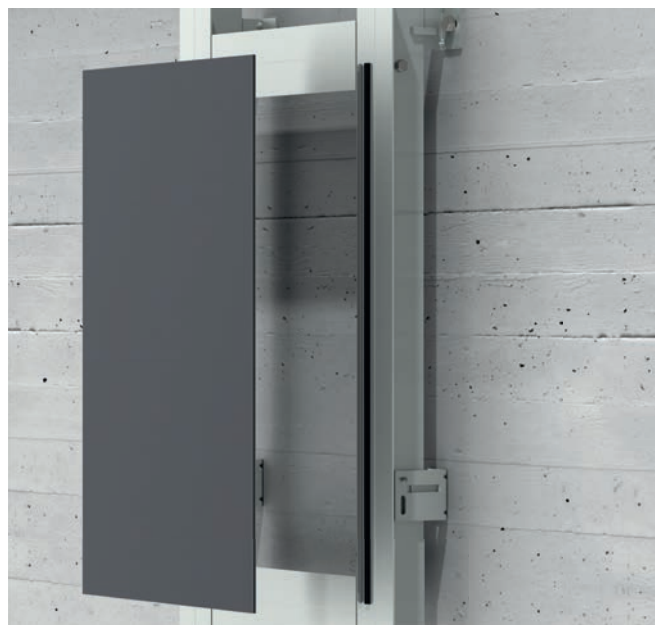
GLUING THE STACBOND COMPOSITE PANEL
