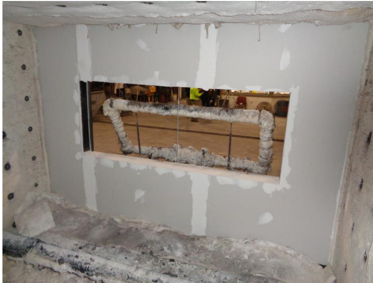
Photo No. 5 Interior Wall Surface First Floor
