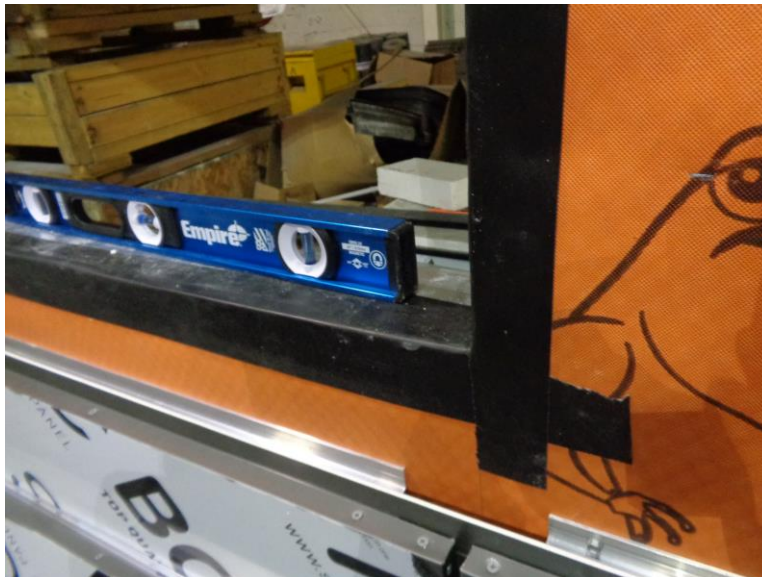
Photo No. 2 Air Vapor Barrier and Window Tape Installed
