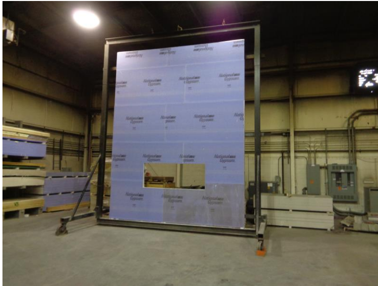
Photo No. 1 Core Wall and Sheathing Installed
