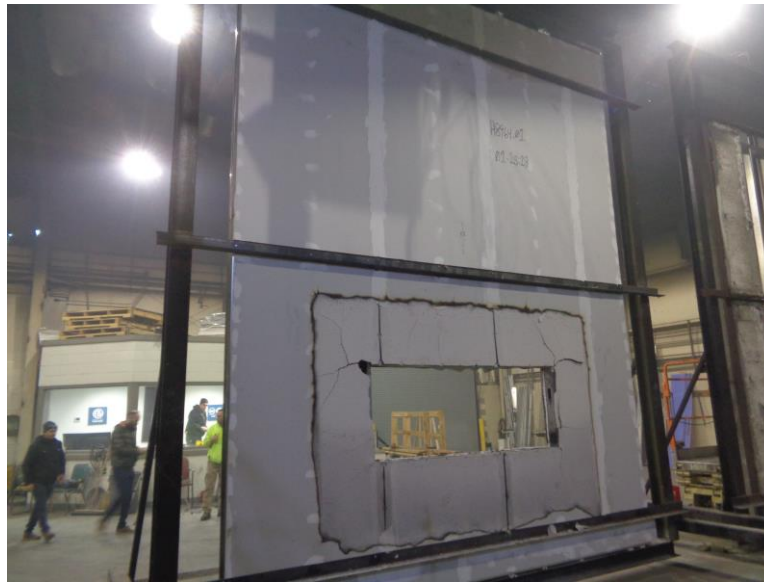
Photo No. 11 First and Second Floor Interior Wall Surface
