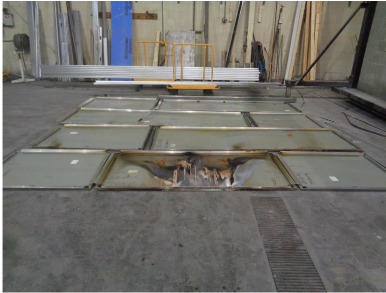
Photo No. 13 Back of Panels
