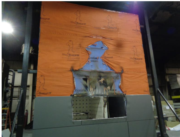
Photo No. 12 Panels Removed
