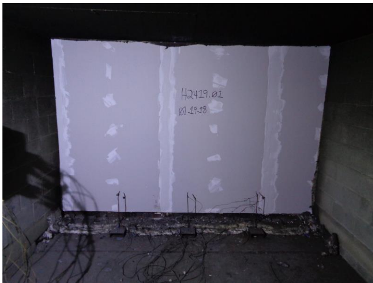
Photo No. 6 Interior Wall Surface Second Floor
