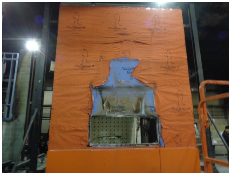
Photo No. 12 Panels Removed
