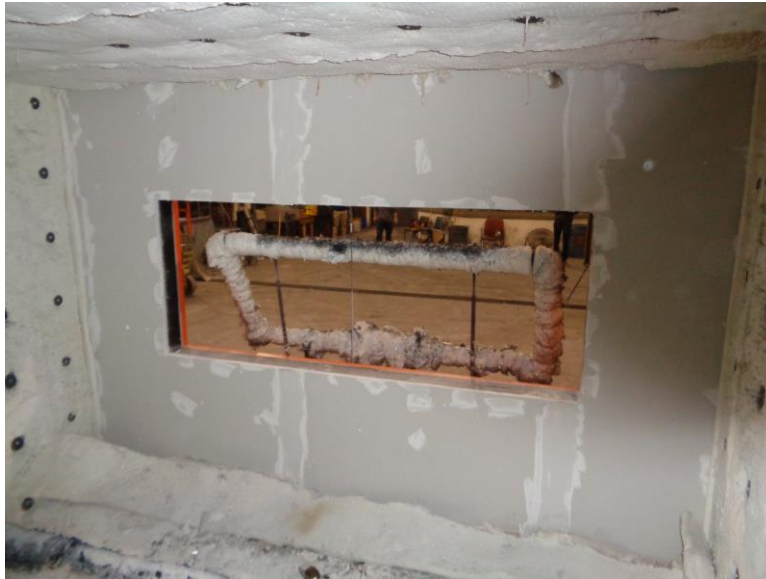
Photo No. 5 Interior Wall Surface First Floor
